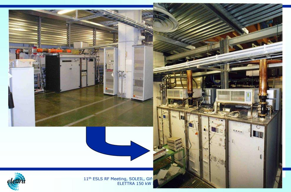
The 150 kW amplifier is made combining two 80 kW IOT transmitters.
