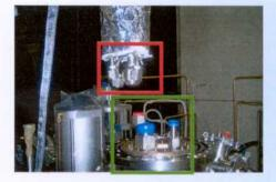
Due to a construction error, the lines in the multichannel line didn't fit to those on the cryomodule. This was discovered after installation, on the 30/08/02.
