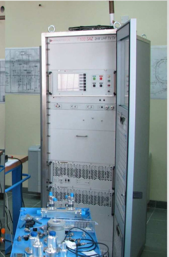
The new 2kW Solid-State amplifier as replacement for the old klystron used in BESSY1
