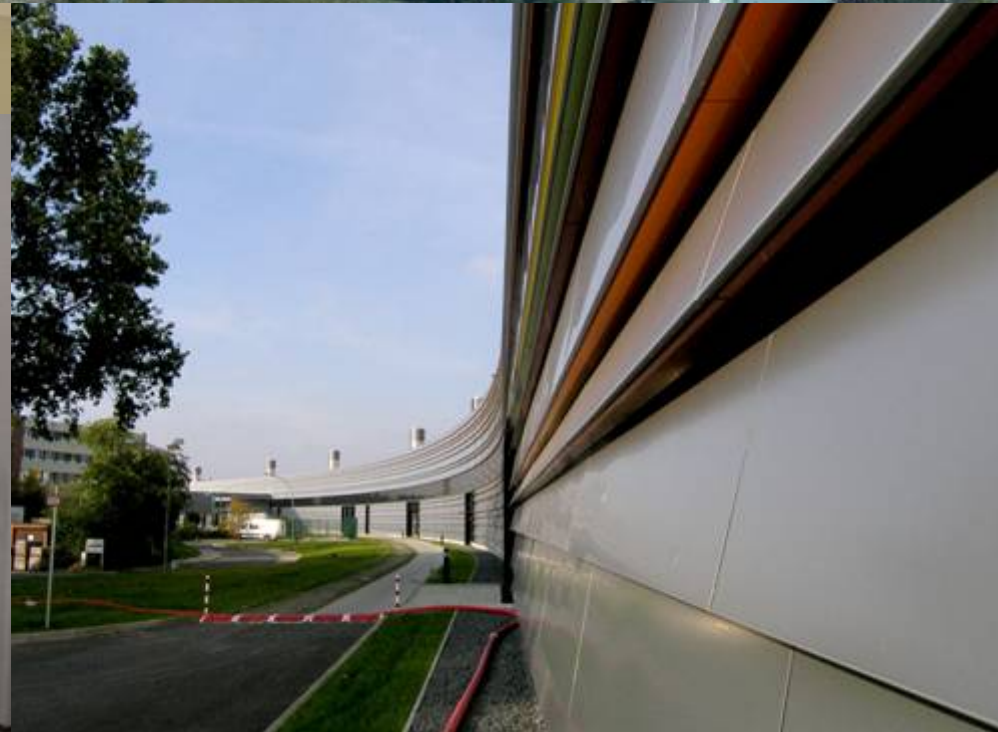
one of 34 moduls on girder
