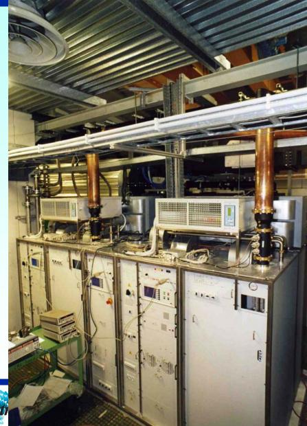
The 150 kW power amplifier is made combining two 80 kW transmitters.
