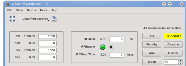
Figure 1: Commissioning FOFB GUI.
